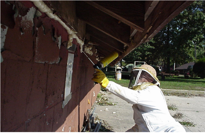
Figure 1.9 Foaming a wall void to exclude yellow jackets.
